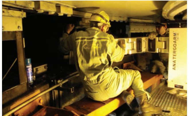
Hydro-Quebec used Robotics Design’s ANATERGOARM to repair and replace 300 kg break units at its Robert Bourassa Generating Station.
